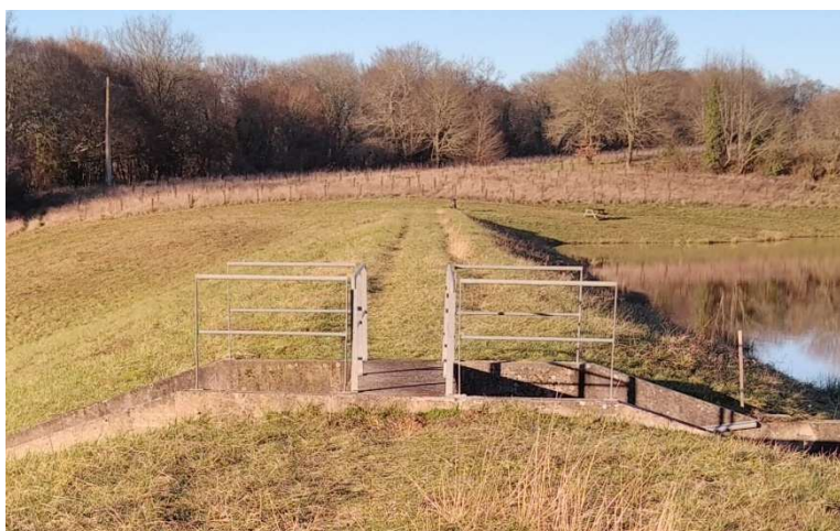
Figure 14 : Barrières garde-corps non conformes
